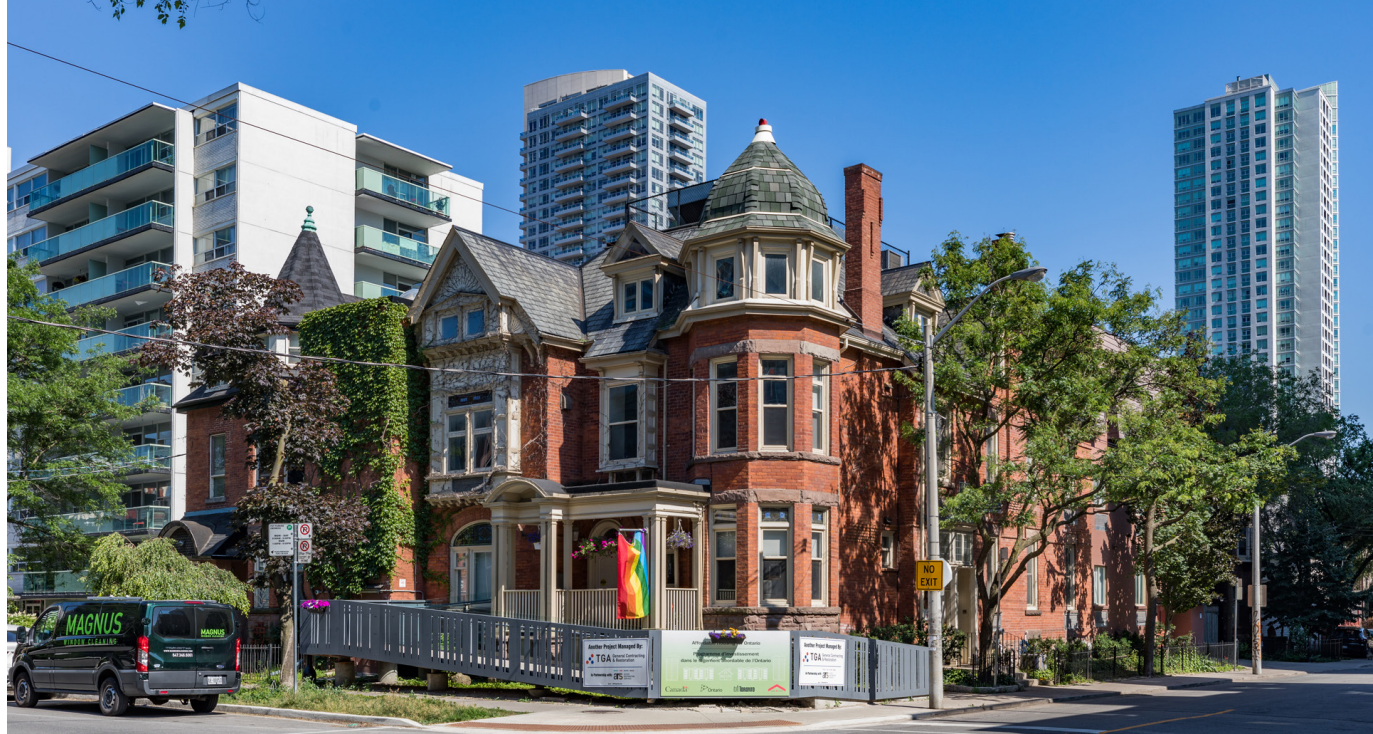
A wheelchair ramp offers accessibility to the Fife House, a historic renovation near downtown Toronto that provides services to people with HIV/AIDS who are also experiencing homelessness.
