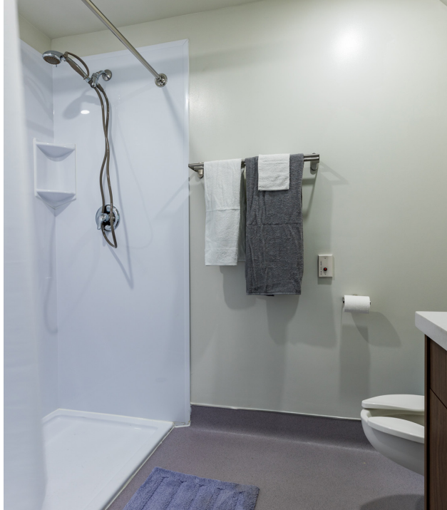
Vinyl and grout-free showers and floors limit the growth of mold and mildew.
